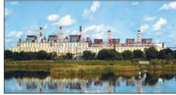
Koradi thermal power station is one of the industries that earned a five-star rating.
